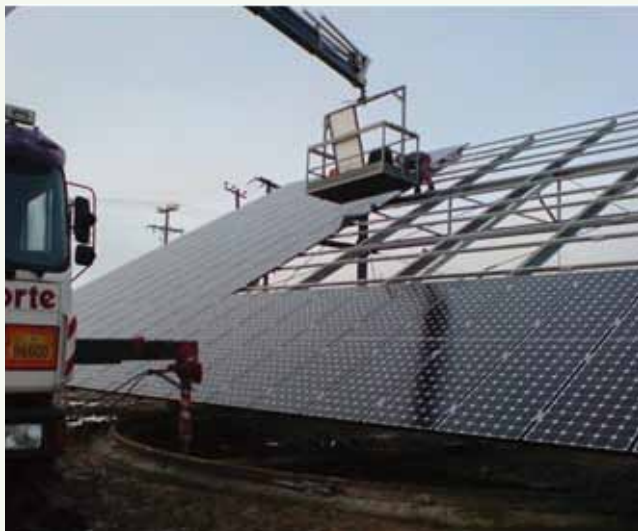
Figure 23: Module Installation on a Large Tracking System
