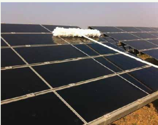
Figure 26 : Module Cleaning Using Dust Broom
