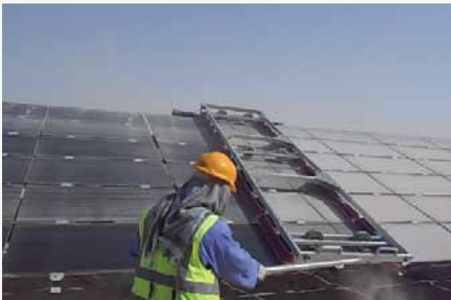
Figure 25: Module Cleaning Using Brush Trolley
