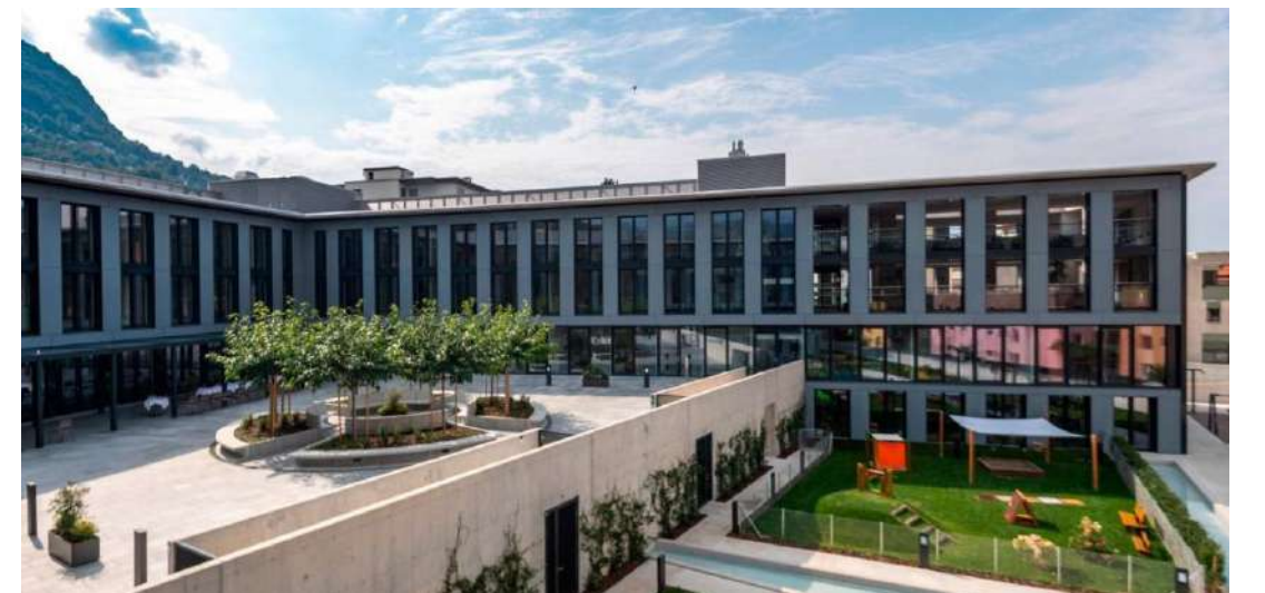
Fig. 3.1 A multifunctional BIPV building in Pregassona, in addition to the home for the elderly, this multifunctional centre in Pregassona houses a kindergarten. Photo credits: Chiara Zocchetti – CdT.
