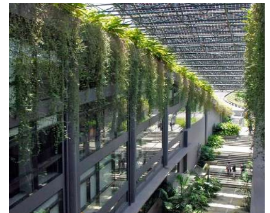
Fig. 4.15 Canopy, interior view. Source: Stapati.
