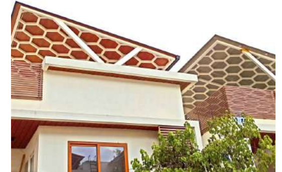
Fig. 4.8 View of the PowerRoof. Source: SunEdison.
