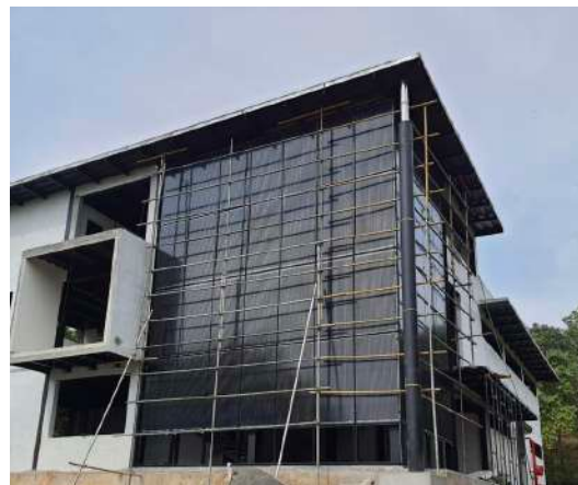
Fig. 4.11 Curtain wall under construction. Source: TopSun
