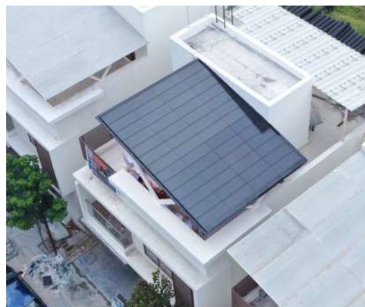
Fig. 4.7 . Aerial view of the PowerRoof. Source: SunEdison
